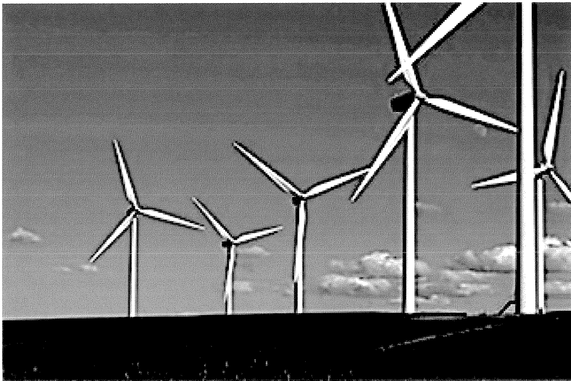
Marengo Wind Project, Dayton, Washington
